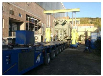
Unloading a transformer with 220 tons
